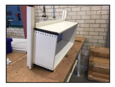
Make sure the frame is pressed horizontally and smooth in the wall opening. Then secure the frame to the wall with (6) screws through the flange in the locations pointed out below. Ensure these screws are sunken into the flange on the upper and lower side so the slide won't hit the screws when opening.
