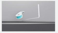
**Step 6.** Install winch block or pulley at the top of the inlet.
