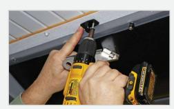
Install winch block for pull wire and rope to go through.
