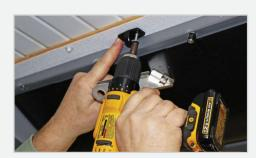
Install winch block for pull wire and rope to go through.
