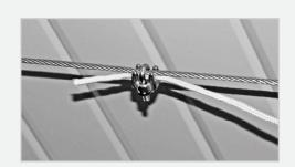
Fasten pull cord to pull wire using cable clamp.
