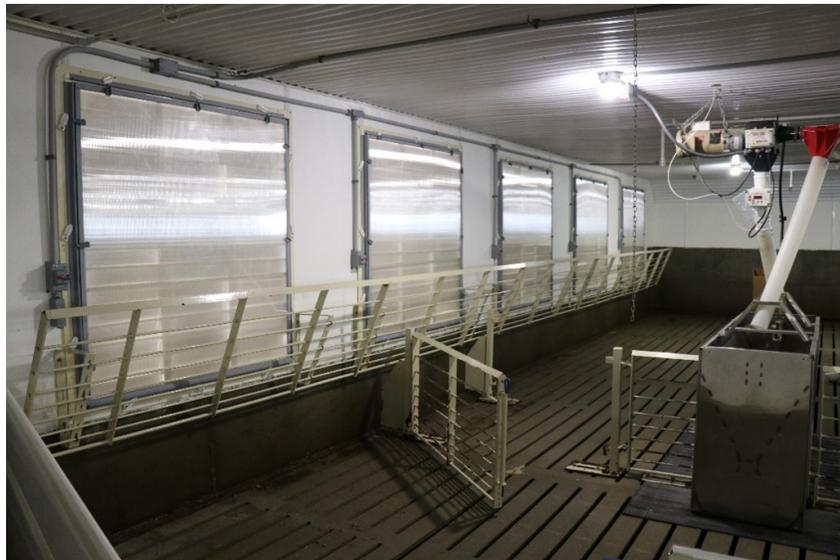
Double L shutter blank installed in a pig barn.
