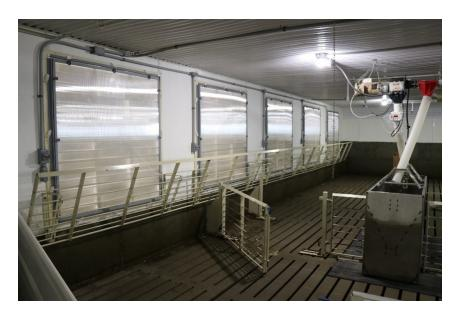
Double L shutter blank installed in a pig barn.
